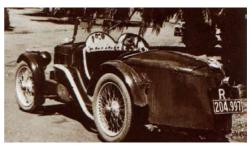
A specially developed twin plate clutch transferred power to the hefty ENV four-speed crash gearbox and the final drive was through straight cut bevel gears. The chassis frame was straight and parallel steel channel which under slung the rear axle and swept over the front axle. Cross-braced tubes passed through the side members and, fixed with brazed flanges, gave a strong yet flexible structure.
