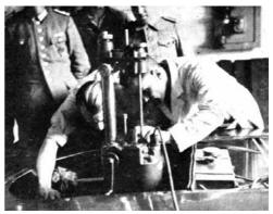
Sid Enever (right) and Reg Jackson boring out the engine in situ in the Dessau police barracks, to make an attempt on larger capacity class record (1939)
